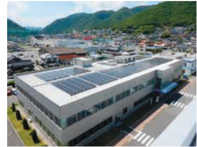
Solar panels at Eagle Industry Co., Ltd.'s Okayama Plant
